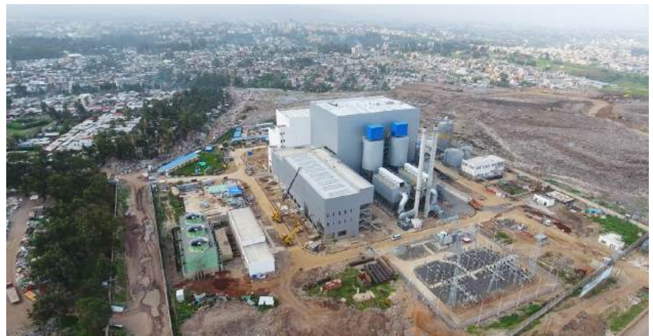
Ethiopia's Koshe Waste to Energy plant
